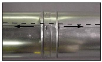
Figure 10.8 Align and Disassemble Vent Sections
